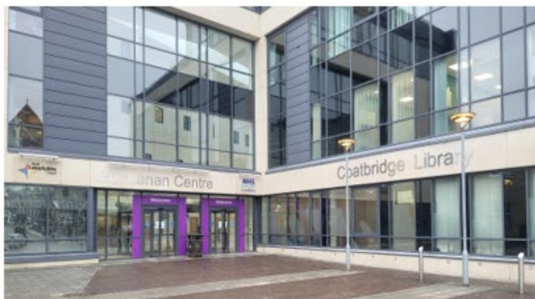
New exterior wayfinding signage, welcome signs and contrasting colour to make entrance clearer. Removal of cluttered signage at entrance.
